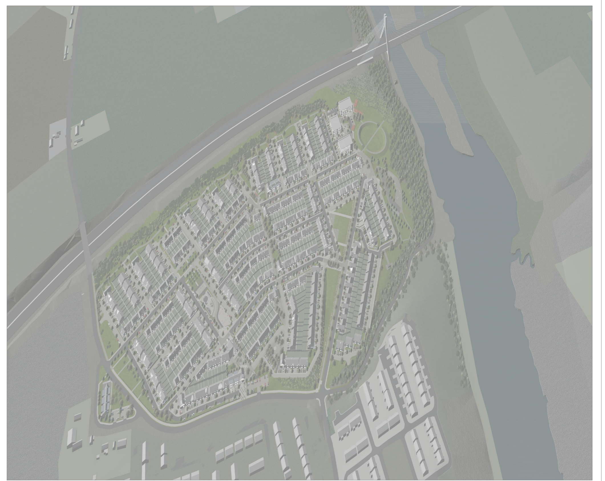
AERIAL SITE VIEW 2 (WEST)
